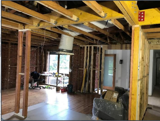
Structural Alteration & Wall Removal
